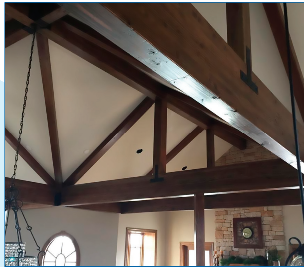
Interior Architectural Beams
